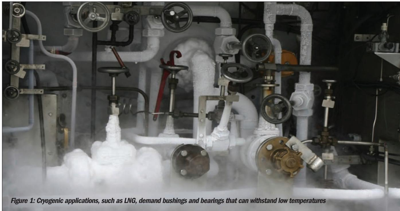
**Figure 1:** Cryogenic applications, such as LNG, demand bushings and bearings that can withstand low temperatures
